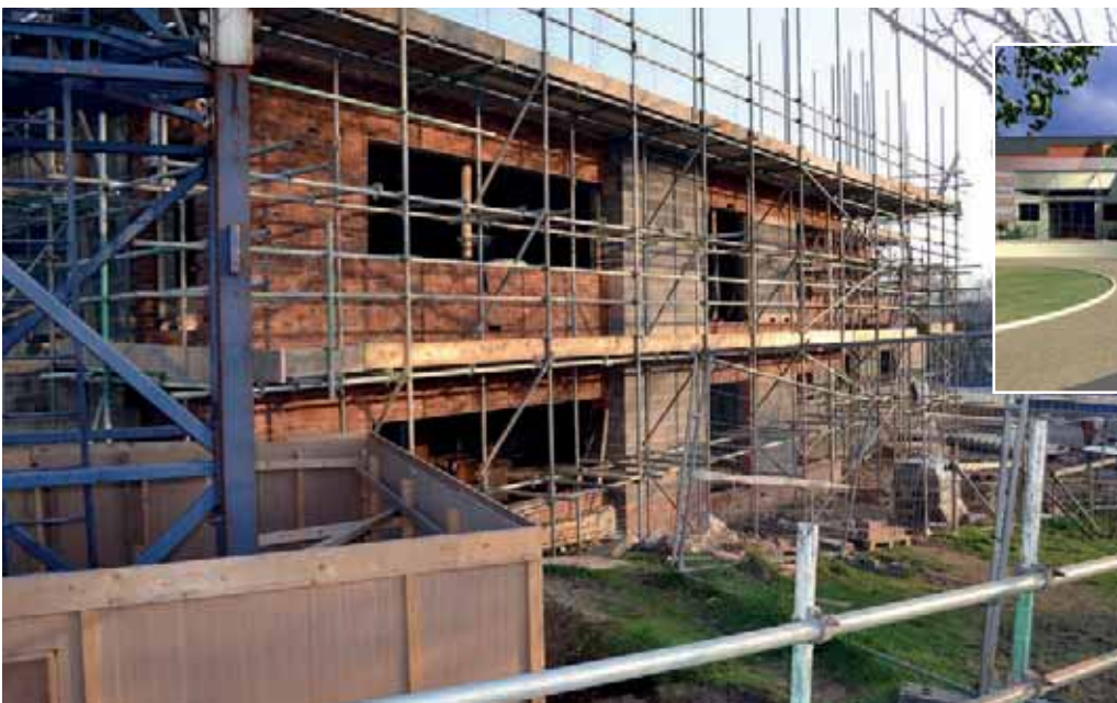
Left The new building is taking shape
